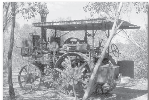
Mallee roller and steam traction engine at Ruedins eucalyptus factory, Bagshot North. Once used to flatten the scrub in preparation for harvesting
