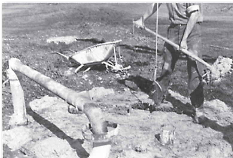
At Ted Hartland's sealing the vat lid with clay and mud
